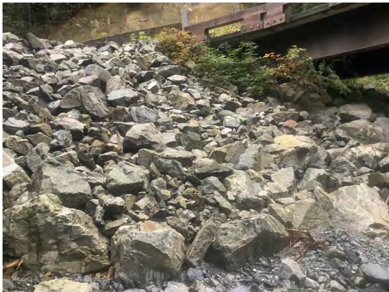
Right Bank Abutment when facing downstream
