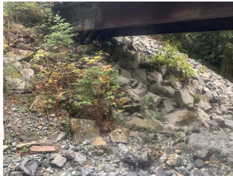
Left Bank Abutment when facing downstream
