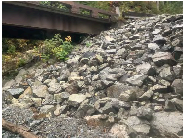
Left Bank Abutment when facing downstream
