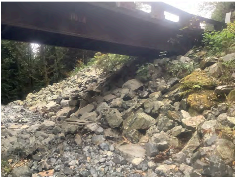
Right Bank Abutment when facing downstream
